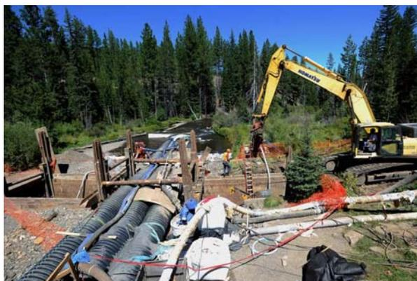
In this 2015 file photo, water from a Tumalo Creek tributary is diverted through a series of large pipes to allow construction crews to install the new Bridge Creek water pipeline last summer. A panel of judges from the 9th Circuit Court of Appeals ruled in favor of the city and the U.S. Forest Service in a lawsuit filed by Central Oregon Landwatch and WaterWatch of Oregon in 2013 (Ryan Brennecke / Bulletin file photo)
